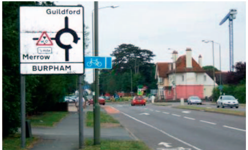
Former Green Man/Harvester pub in the middle of Burpham, prior to demolition by Aldi.
